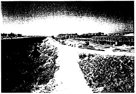
Guadalupe River Flow - Low/Low Tide August 1997 Looking Downstream from Tasman Ave. Bridge Development Next to Levee, Ground Floor of Housing is Below the High Tide of the River
